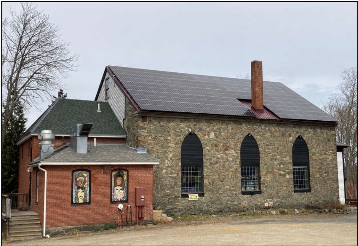
The historic Stone Church on Zion Hill- 25.92kW array and EV charging station installed by ReVision Energy in July 2019
