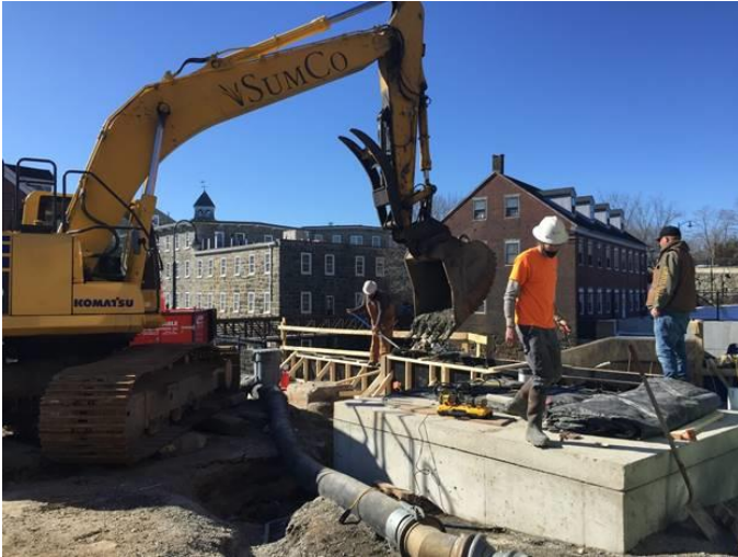
SumCo placing concrete for the curb wall
