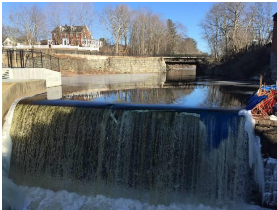
Flow over the main spillway
