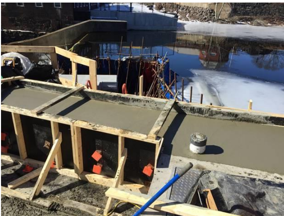
Applied concrete finish of the curb wall
