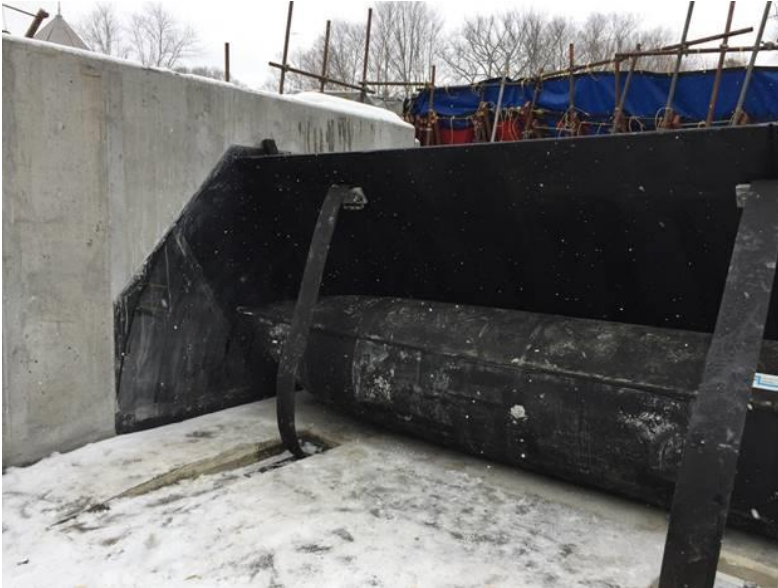
Installed tension straps.
