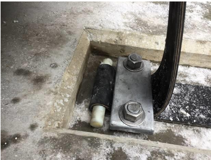
Tension strap anchor plate in the tension strap cutouts of the spillway
