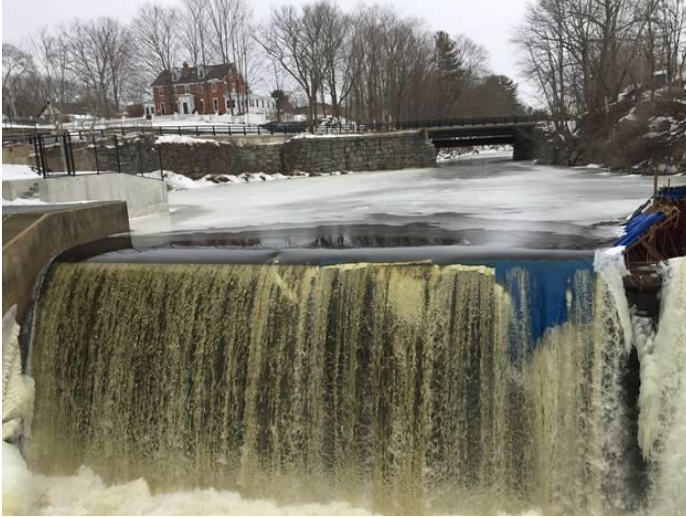
Water flow over the main spillway
