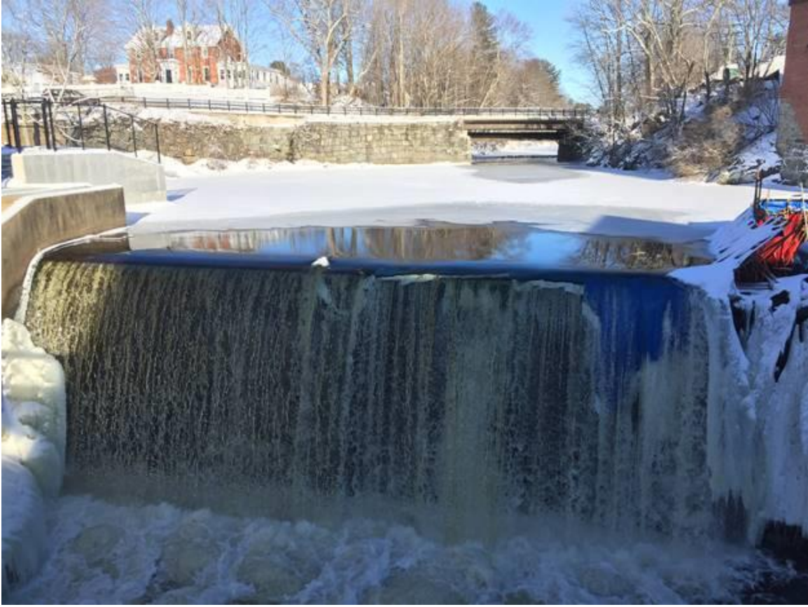
Water flow over the main spillway
