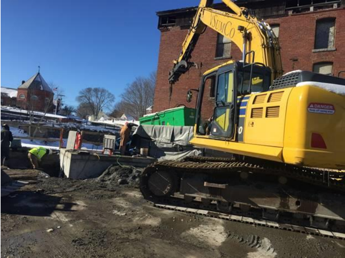
SumCo moving the pump to its original location
