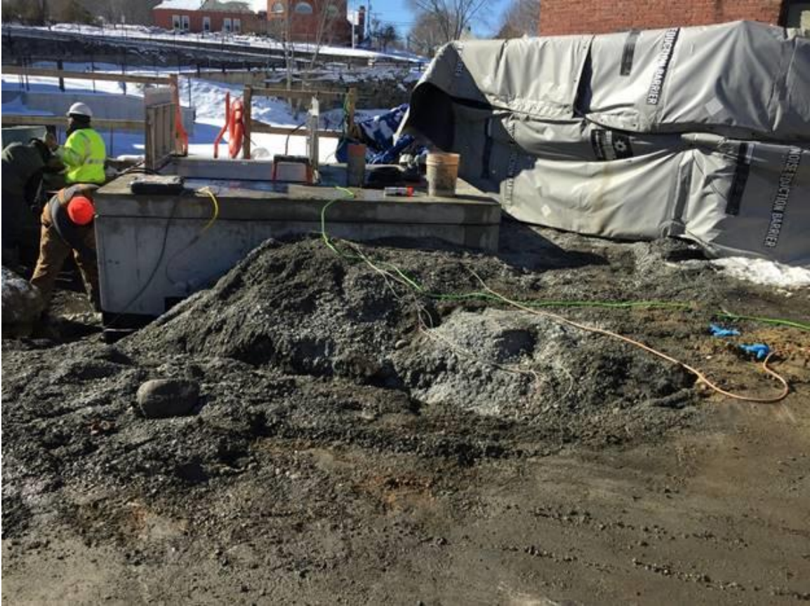
Uncompactd lift of crushed gravel placed around the vault.
