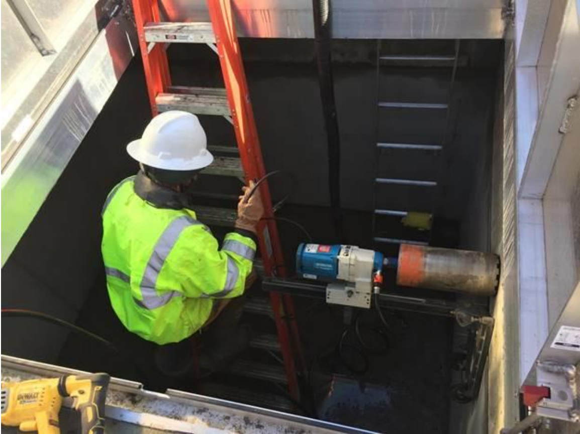
SumCo coring conduit holes in the vault
