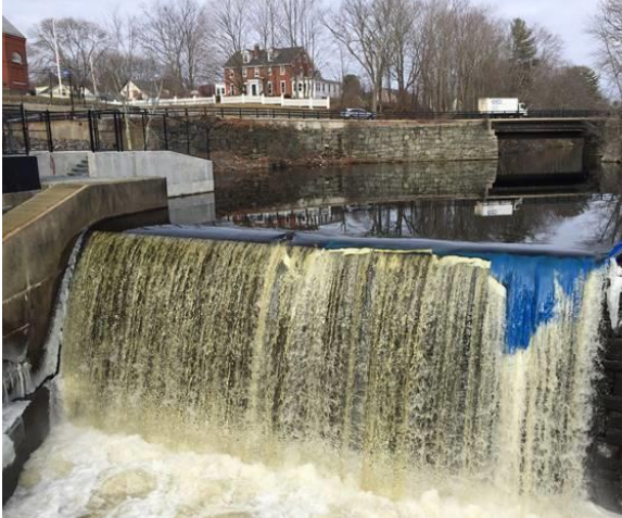
Water flow over the main spillway
