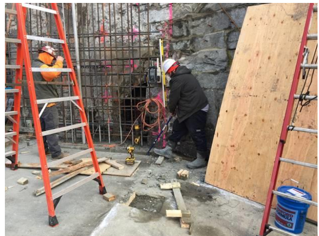
SumCo removing wood forms from around the East abutment wall
