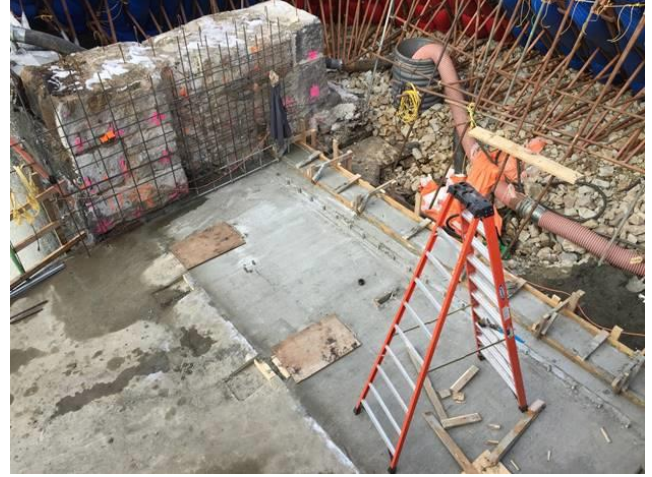
Gate footing area
