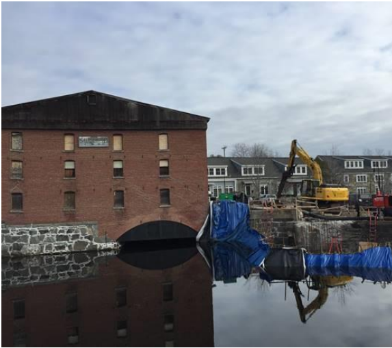
View of the Portadam from the right abutment area
