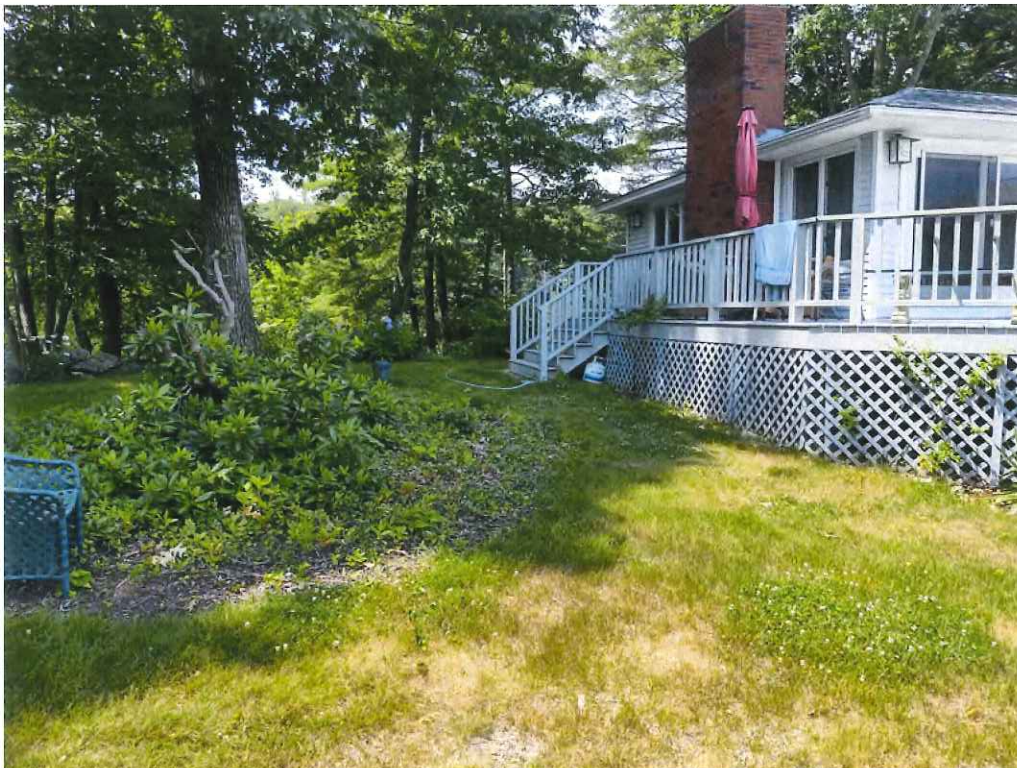
4. Looking west at the proposed location of the addition.
